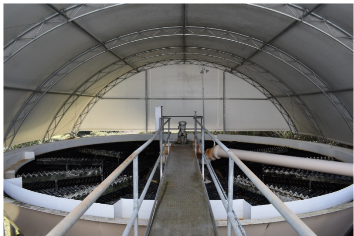
SDC Water Treatment Plant
